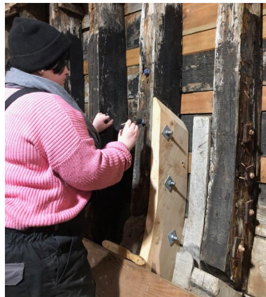
Treating exposed metal with rust converter
