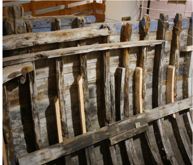
New wooden clamps to reinforce the frames
