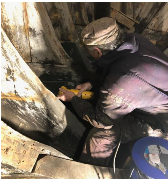
Fitting new bolts to the frames
